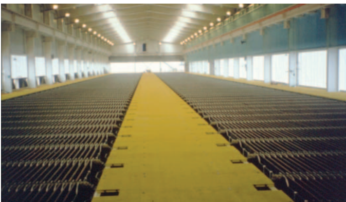
Copper processing facilities such as the Ammonia Leach/Solvent Extraction/Electrowinning plant for Minera Escondida Limitada in Chile found DURADEK® I-6000 1-1/2" to be the perfect solution.
