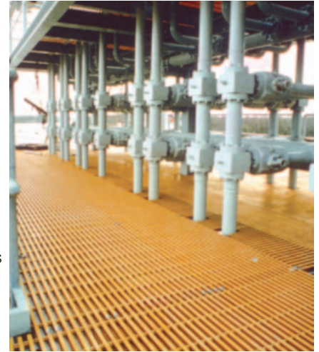
DURAGRID® Phenolic grating was used on Shell's Mars offshore platform for fire integrity, weight savings and low maintenance. DURAGRID® Phenolic is U.S. Coast Guard approved.
